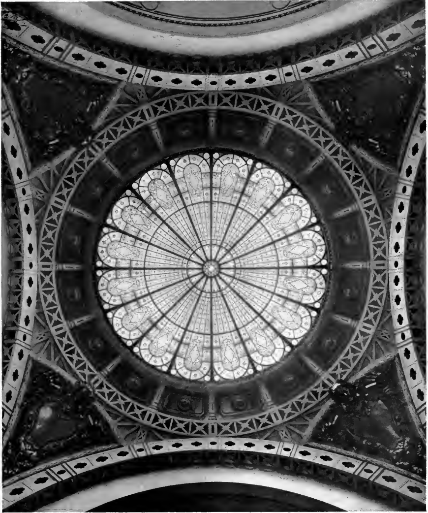
DETAIL OF THE DOME. (The National Park Bank.)
